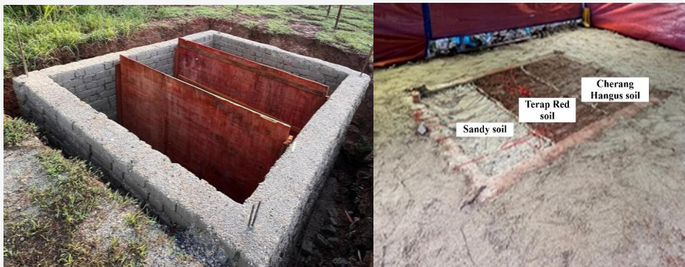
Figure 2: A simulation leachate tank of 3.0 x 2.5 x 2.0 meters and 5 cm in thickness
