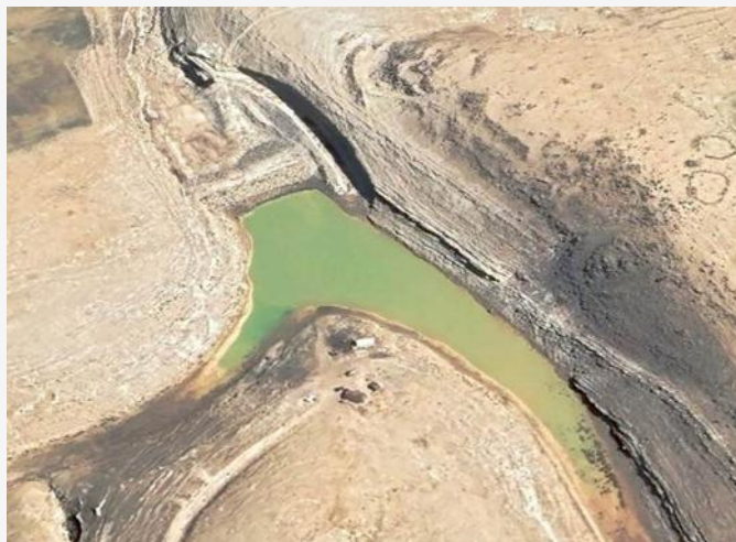
Figure 1: Hamoud check dam in the Al-Mujib Basin
