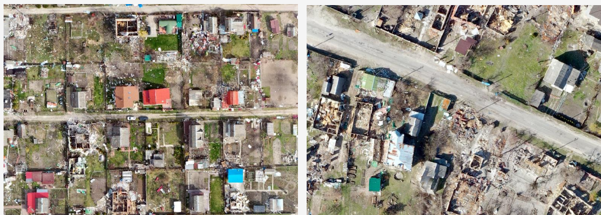
Figure 15: Enlarged fragments of the orthophoto plan showing the scale of destruction to civilian structures
