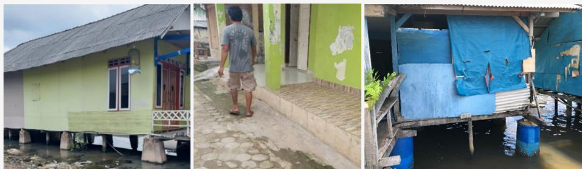
Figure 7: Community adaptation by raising the house building in Bandar Lampung City coastal area
